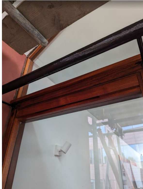
External view of trickle vent
