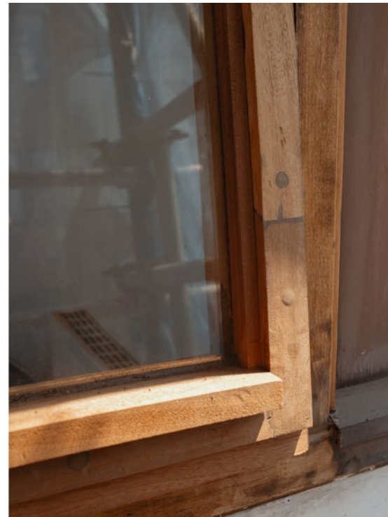
Window repaired with new sapele spliced into frame
