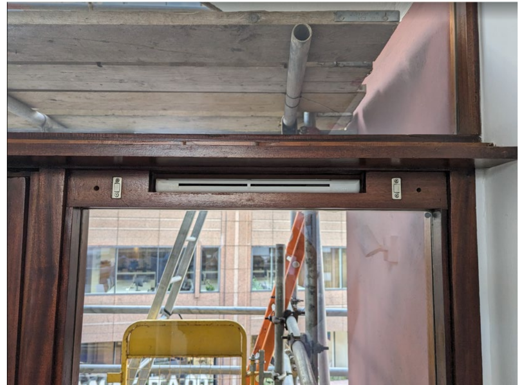
Trickle vent with sapele cover removed
