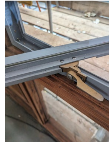
Existing window with VIG installed
