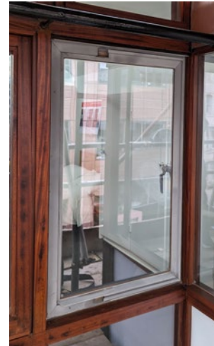
Existing window with VIG installed
