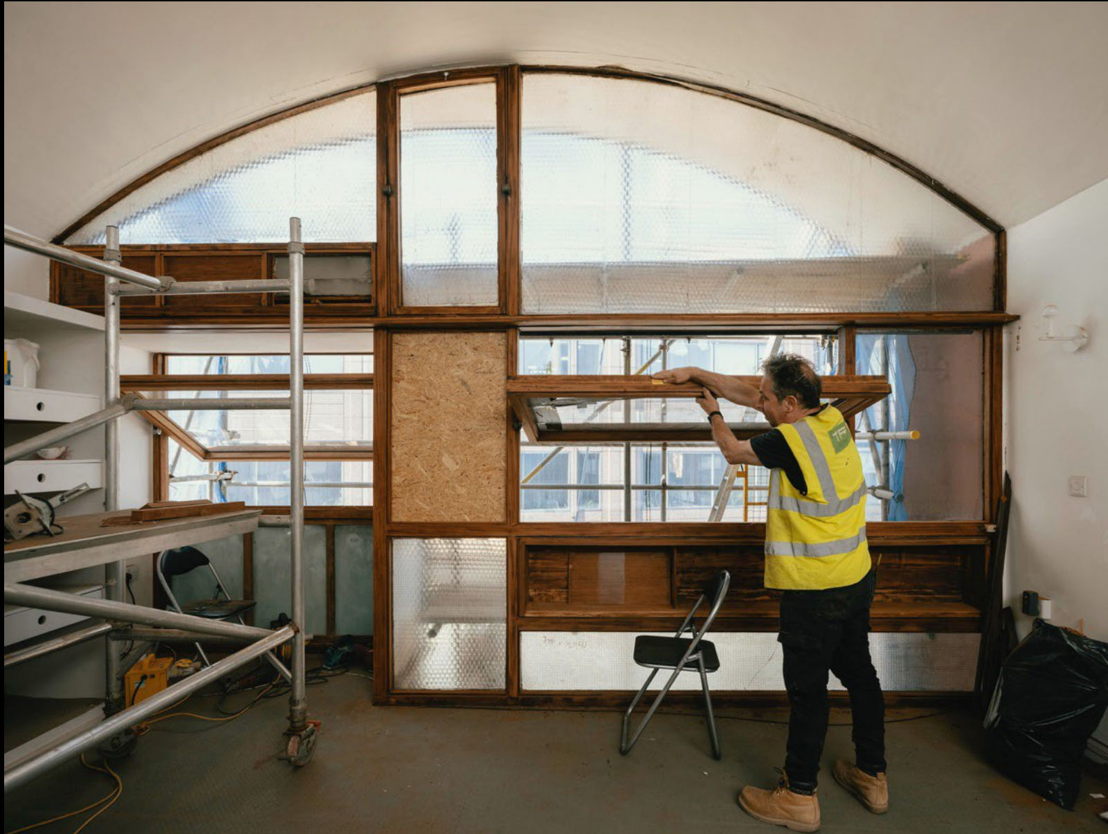
Interior of 347 Crescent House during Pilot Project
