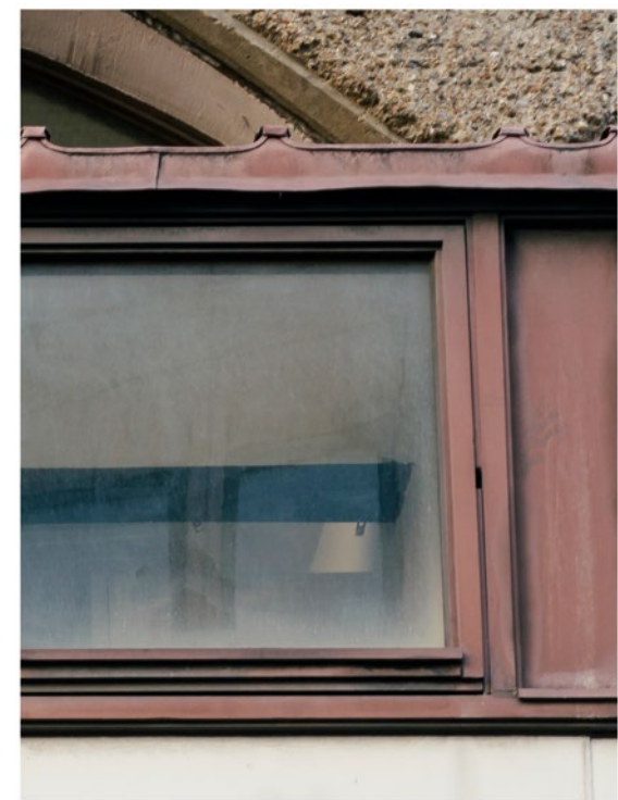
Original Window – no obvious rot
